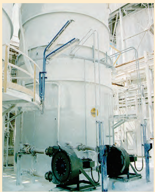
Expensive chemicals and compounds, including adhesive resins, polymers, and latex are protected by Vector pumps during processing.
