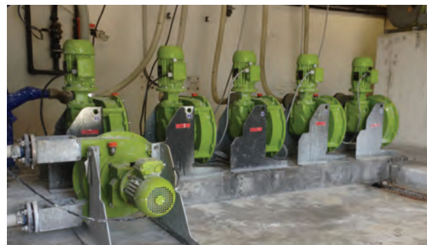
ALHX40 for lime milk in wastewater treatment
