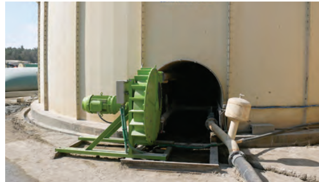
ALH100 pumping thickener underflow in a quarry
